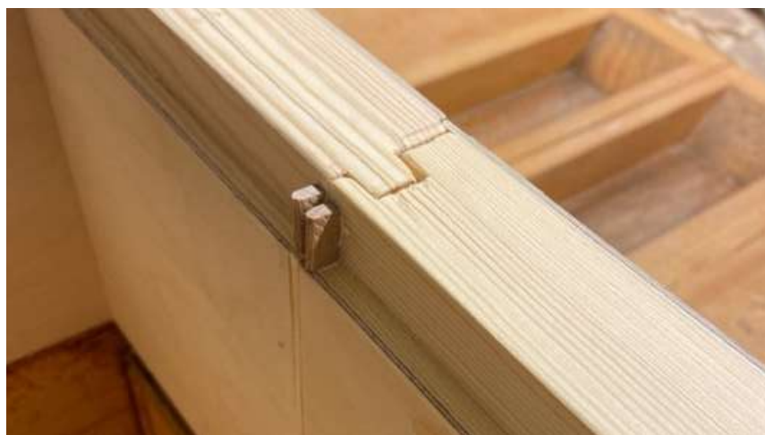
Figure 28: Stops preventing frames from falling out.
