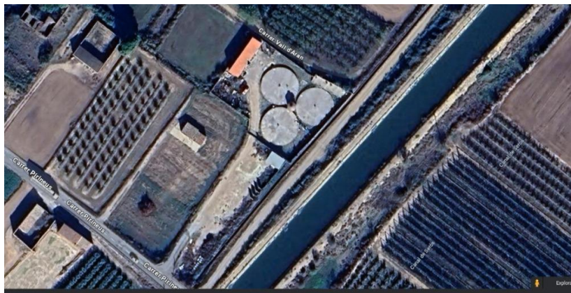
Image 2: Municipal Torres de Segre plant
